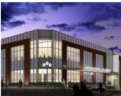
SARATOGA SPRINGS CITY CENTER
